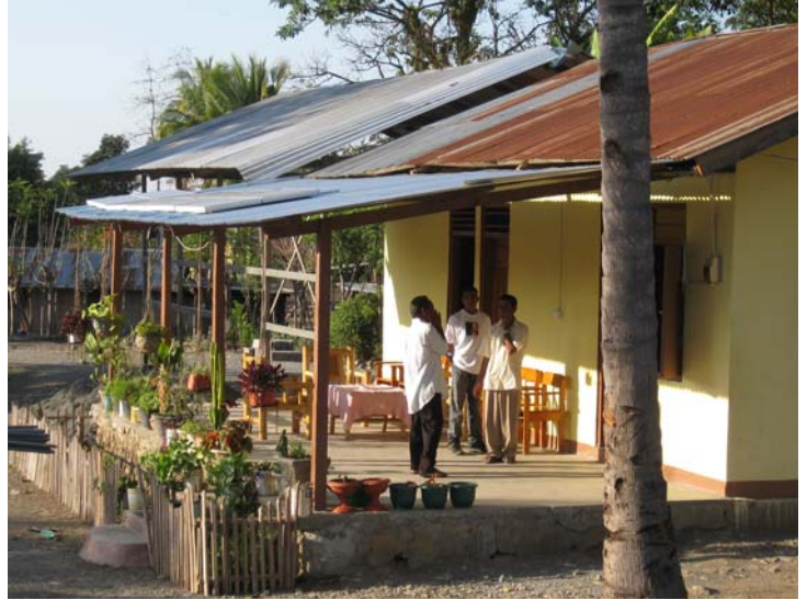
Solar Panels at the Zumalai Compound
