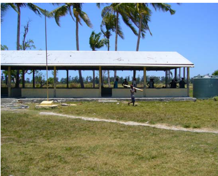
The old school building with the windows and doors gutted
